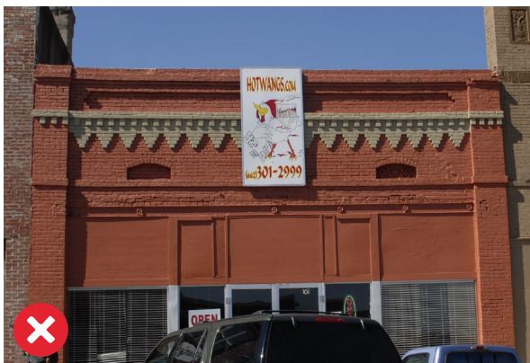
All signs should respect and complement the architectural details of the building. Signs that overlap brick details should be discouraged.
