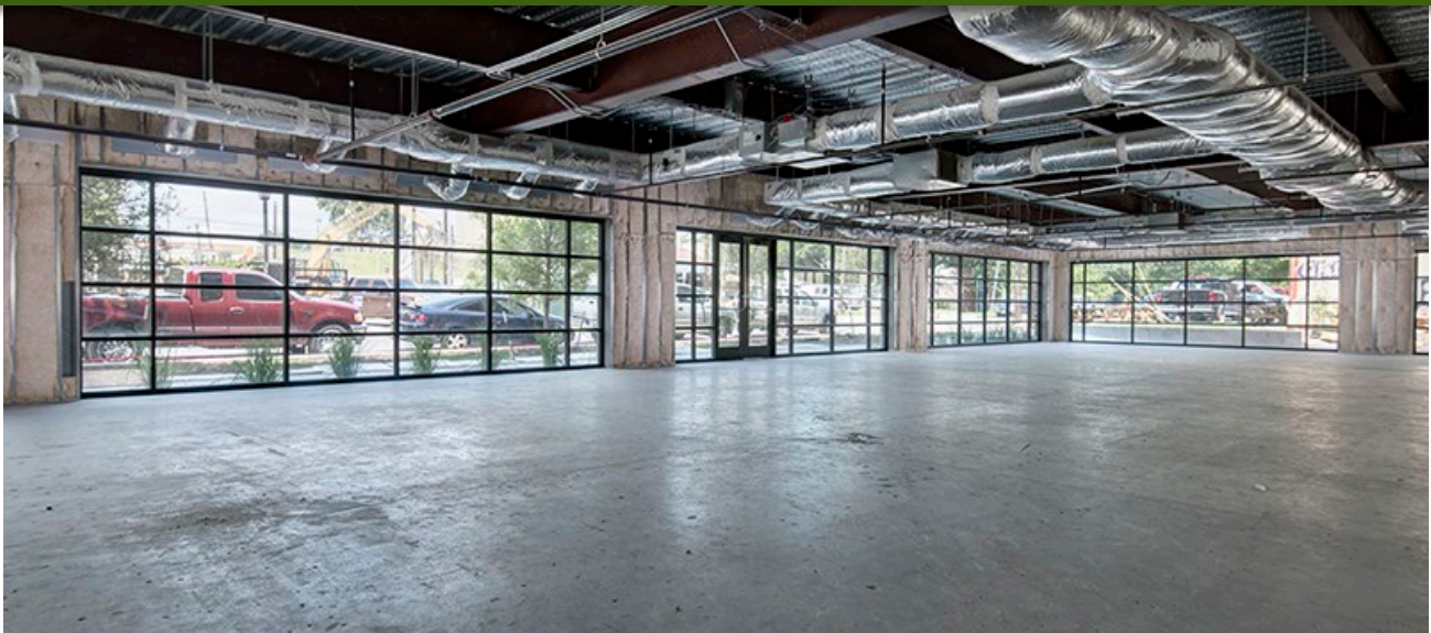
A typical example of a shell space in a new development
