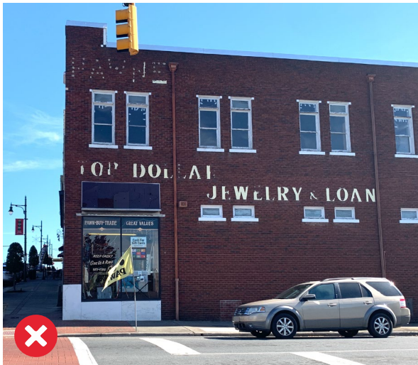
Broken and missing signs create a negative impression for visitors.
